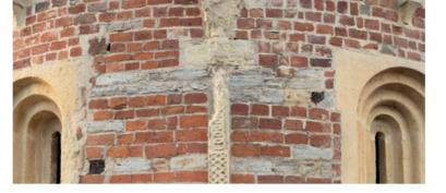
state of deterioration; infiltration of rain water had caused the roof to collapse, together with the vault of the first span over the hall; vegetation had penetrated the walls and caused damage and detachment of some of the decorative stonework on the upper cornice. After inspection by the Superintendency in 1984 and subsequent careful restoration and consolidation, under the care of an architect (Inzerra), the building regained its original dignity in the early 1990s.
