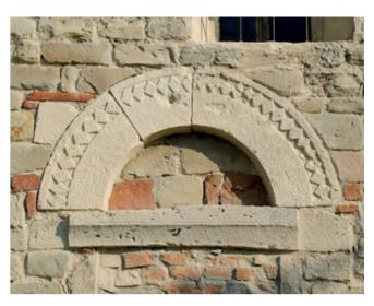
recycling the original dressed stones, material which is exactly like the base. The north side and the façade underwent work in the seventeen hundreds. In the north side, though, a large trapezoidalshaped dressed stone can be seen, which might have belonged to the Romanesque entrance doorway.
